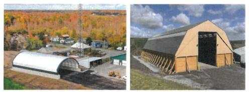
B&L designed and provided construction administration and periodic site inspections for sand and salt storage facilities located in the towns and counties listed. The fabric roof style buildings are generally 37 feet high by 72 feet wide by 90 to 180 feet long with cast-in-place reinforced concrete push walls. These facilities store approximately 7,500 tons of product.
